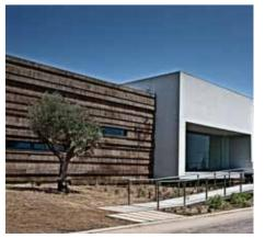
Expanded insulation cork board, a 100% natural material for sustainable construction
